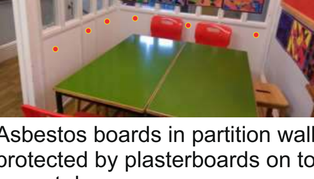
Inspection point n 33
