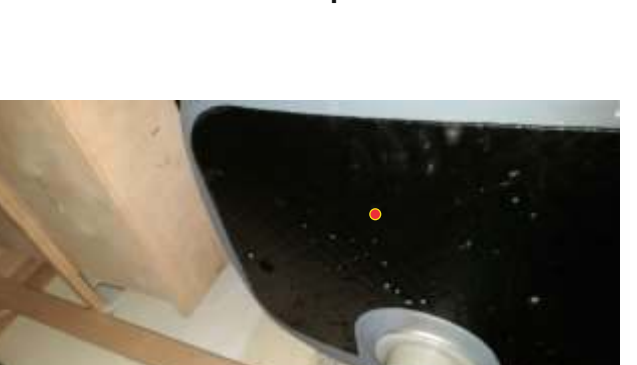
Inspection point n 31
